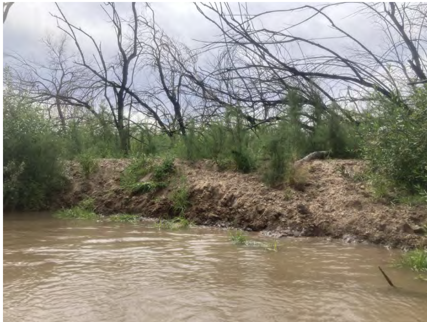
Hoof damage to banks by unauthorized cattle in southwestern willow flycatcher and yellow-billed cuckoo critical breeding habitat on the Myers allotment, Pinal County, during flycatcher breeding season. 33.090026, -111.195096. April 12, 2023.
