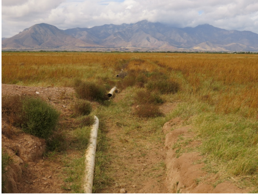
Photograph #13. This photograph is taken from the wellhead for the agricultural well in the southeast quarter of the section, looking west to the Huachuca Mountains. There is an open ditch in the area with remnants of the eight inch PVC pipe in the bottom.
