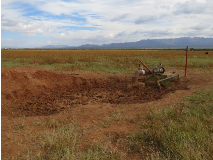
Photograph #7. Photograph of agricultural well distribution system for agricultural well in northeast quarter section, looking east northeast. System remains in place. Precipitation accumulates in the pit that livestock use when grazing. Electrical power was in pipe laying down to the south of the distribution system.
