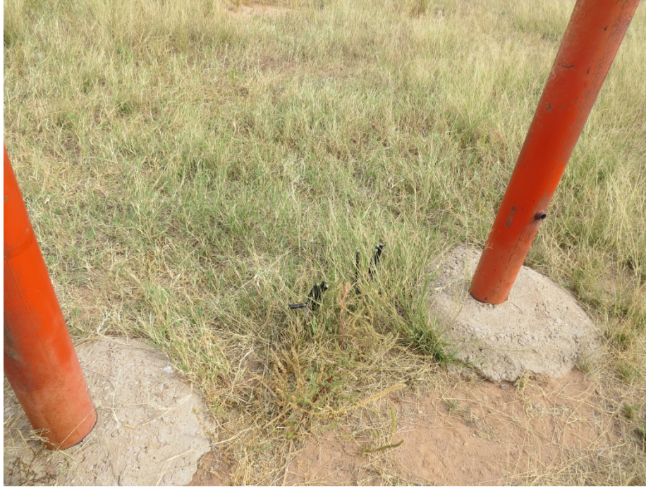
Photograph #5. Power lines to the wellheads and then to the center pivots were located in the ground between the two orange poles shown in Photograph #4 above.
