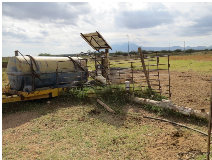
Photograph #2. The first wellhead is located closely adjacent to the entrance gate. There is a submersible pump in the well head that pumps water to the water wagon for distribution to three livestock tanks. View is looking to the southeast from the northwest side of the wellhead.
