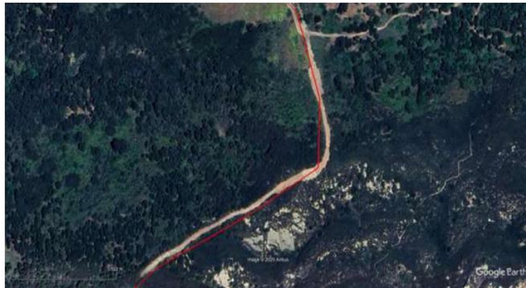
Fig. 1b. Same area on 22 May 2025 showing significant vegetation removal and grading along access road.
