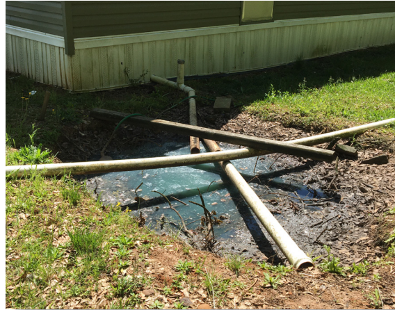
Straight piping sewage to ditch behind home in Lowndes County, Alabama. Photo Credit: DOJ/Civil Rights Division
