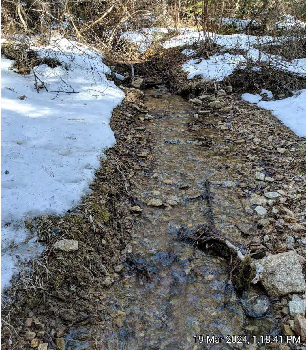
A third culvert removal along reclaimed 5620 on a perennial tributary.
